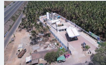
LNG/LCNG fuel stations
